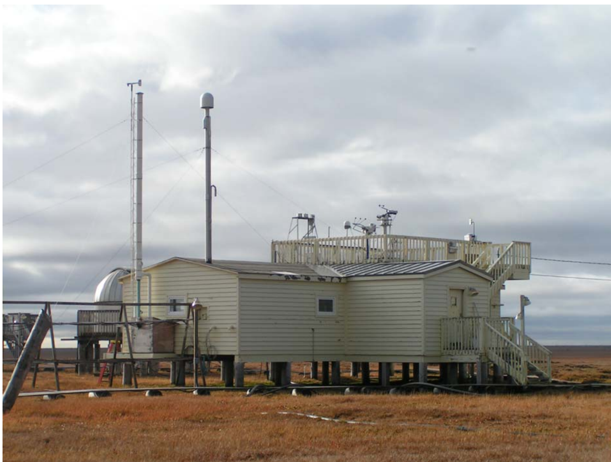
Fig. 1: Outer view of GAW station Barrow, Alaska
